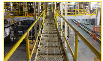
CATWALK GUIDE RAIL
