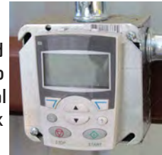
Keypad relocated to 4x4 electrical box
