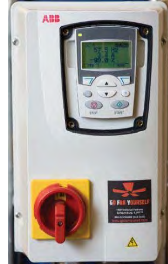
Keypad relocated to 4x4 electrical box
